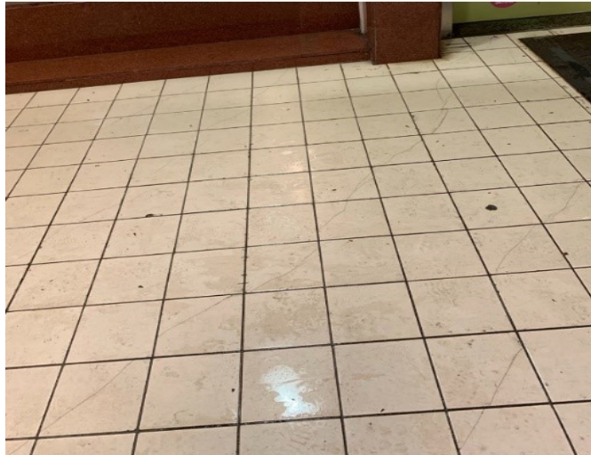
(a) Slab cracking when the seismic condition of a building changes slightly to a non-seismic condition (Hsu, 2022b)
