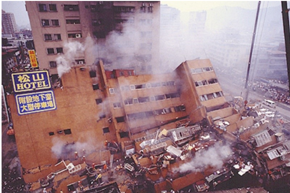
(c) Fall and collapse of a building when the seismic condition of a building changes highly to non-seismic (Zhao, 2020; Hsu, 2022b)
