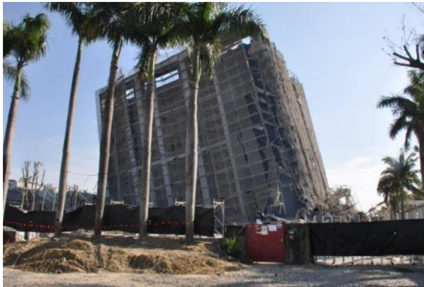
Figure 2. Failure in a building that complied with the latest seismic design code during the 2016 Meinong earthquake in Taiwan (Hsu, 2022a).
